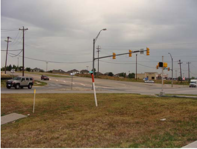
Park Vista Blvd. and N. Tarrant Pkwy intersection (picture taken from median on N. Tarrant Pkwy, looking south)
