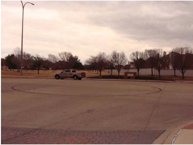
Park Vista Blvd. at Ash River Rd. intersection
