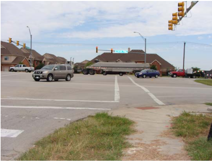
Parkwood Hill Blvd. and N. Tarrant Pkwy intersection (picture taken from Parkwood Hill Blvd. looking north)
